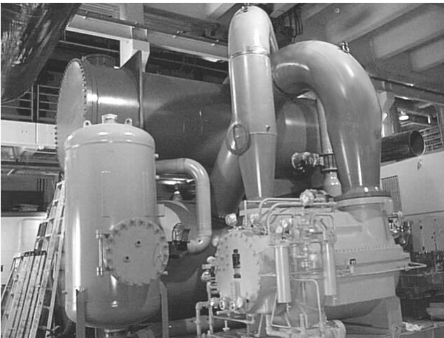
FIG. 14 - MAJOR REFRIGERANT PIPING ASSEMBLY
