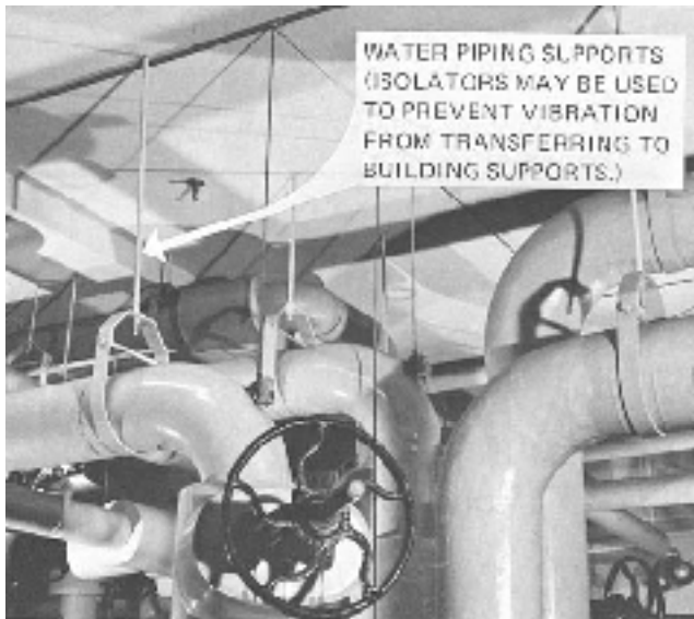
FIG. 17 – TYPICAL EVAPORATOR - CONDENSER WATER PIPING SUPPORTS
