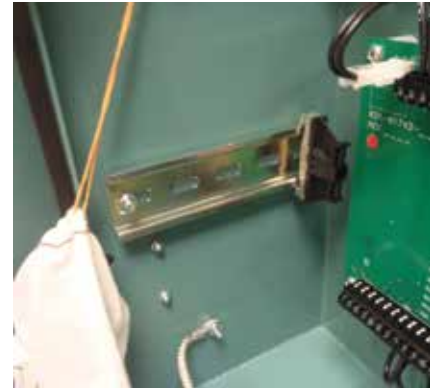
FIGURE 28 - DIN RAIL END BLOCK
