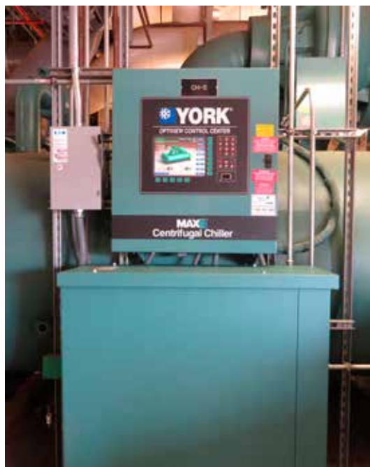
FIGURE 2 - INSTALLATION SHOWING CASL UPS CABINET LOCATED BELOW THE OPTIVIEW CONTROL PANEL
