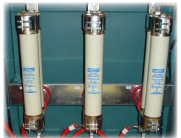
FIGURE 9 - E-TYPE MAIN FUSES
