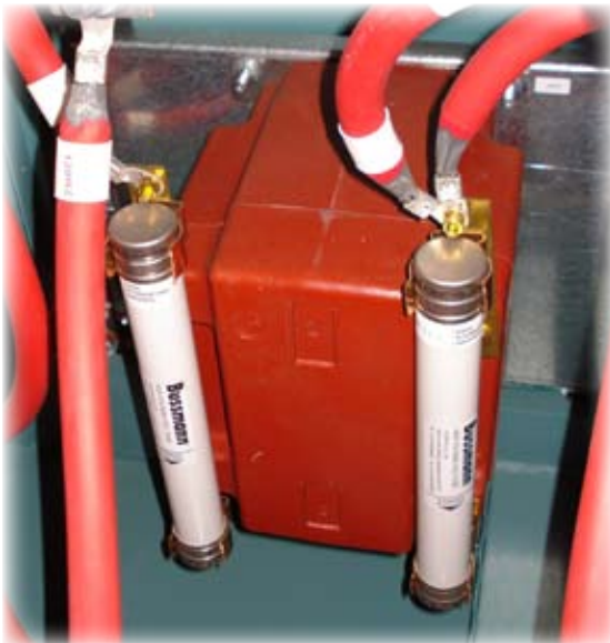
FIGURE 12 - CONTROL POWER TRANSFORMER
