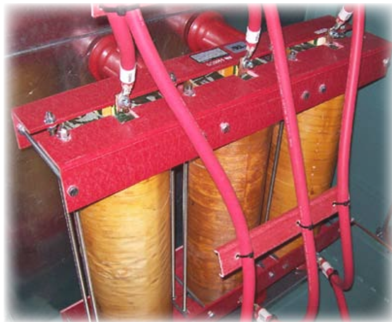
FIGURE 6 - PRE-CHARGE REACTOR
