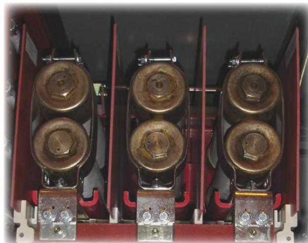
FIG. 9 – E-TYPE MAIN FUSES
