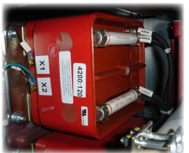
FIG. 12 – CONTROL POWER TRANSFORMER
