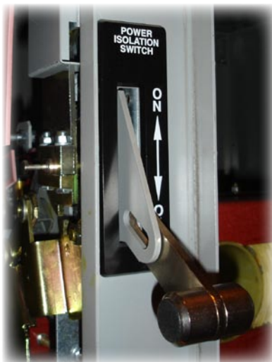
FIG. 10 – ISOLATION SWITCH JOHNSON CONTROLS
