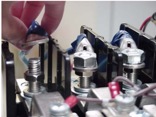
Figure 5-1 Disconnecting the AC Input Cables
