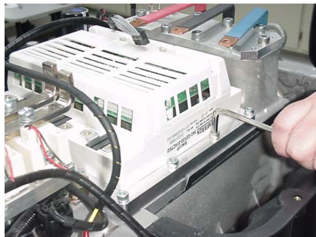
Figure 6-18 Removing the IGBT Inverter
