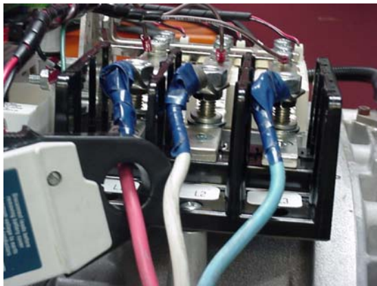
Figure 4-28 Phase Current Measurement
