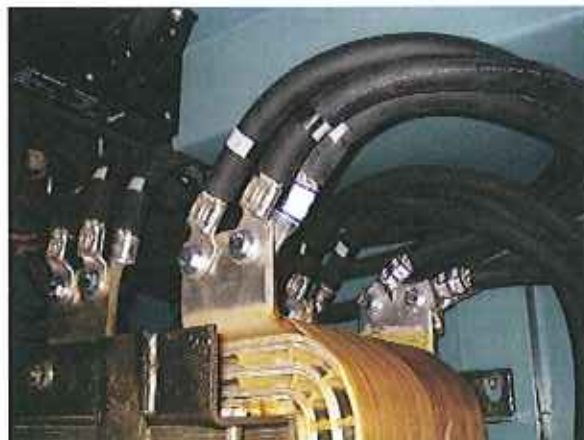
Modified 1L Inductor is Moved into Position
