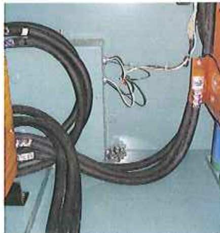
New Wires are added between 1L and DC bus
