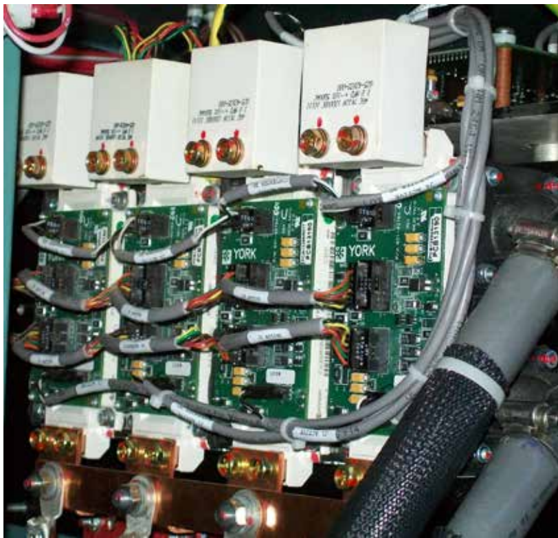
FIGURE 11 - RECTIFIER SIDE OF THE POWER UNIT (MODEL 744 SHOWN).
