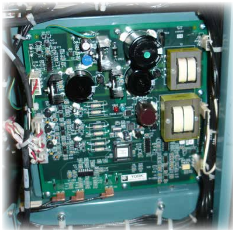
FIGURE 3 - SCR TRIGGER BOARD
