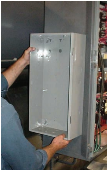
Figure 16. Mounting starter sub-box
