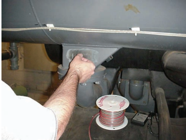
Figure 11. Sensor mounting with Armaflex insulation
