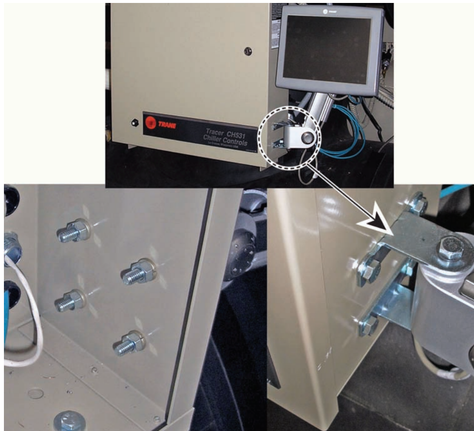
Figure 6. Bolting display arm to the panel
