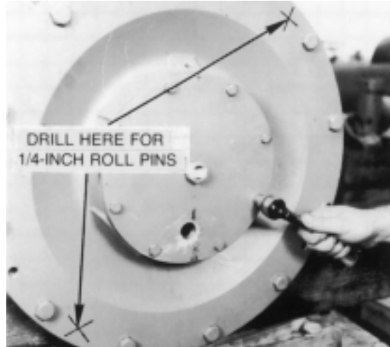
Figure 4. Removing bearing inspection plate
