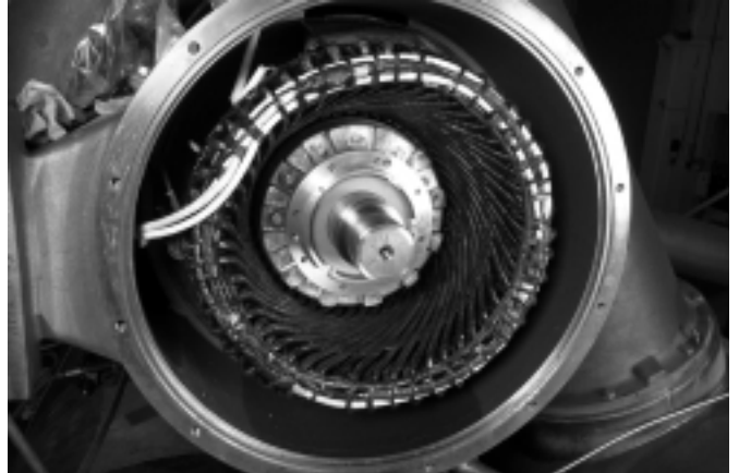
Figure 19. CVHF 1470 or 1720 motor with thrust bearings removed. The bearing cap is shown in place in preparation for a new thrust bearing installation.
