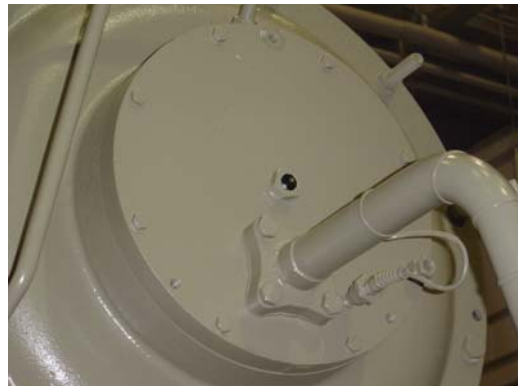
Figure 5. New design Bearing Inspection Cover with brush fitting, but without the brush installed. This cover is standard on LF 2.0 equipped chillers since 9/24/2004.
