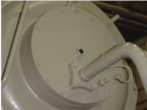
Figure 5. New design Bearing Inspection Cover with brush fitting, but without the brush installed. This cover is standard on LiquiFlo2.0 equipped chillers since 9/24/2004.
