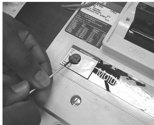
Figure 4: Prying the rating plug
