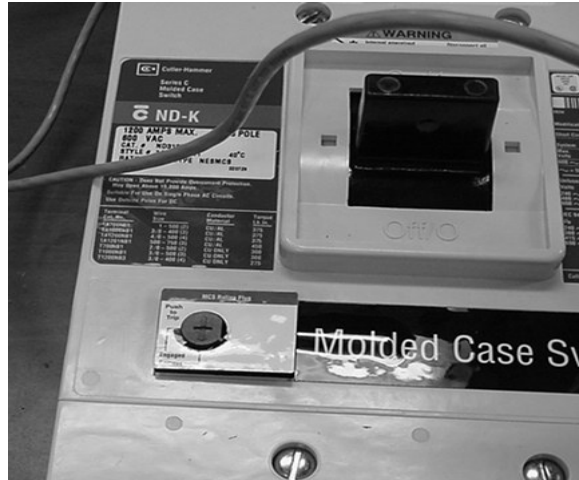
Figure 5: Removing Rating Plug
