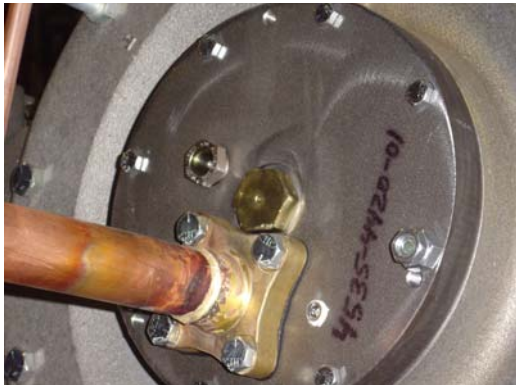
Figure 5. New design Bearing Inspection Cover with brush fitting, but without the brush installed. This cover is standard on LiquiFlo2.0 equipped chillers since 9/24/2004.
