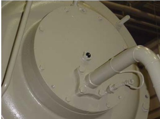
Figure 5. New design Bearing Inspection Cover with brush fitting, but without the brush installed. This cover is standard on LiquiFlo2.0 equipped chillers since 9/24/2004.
