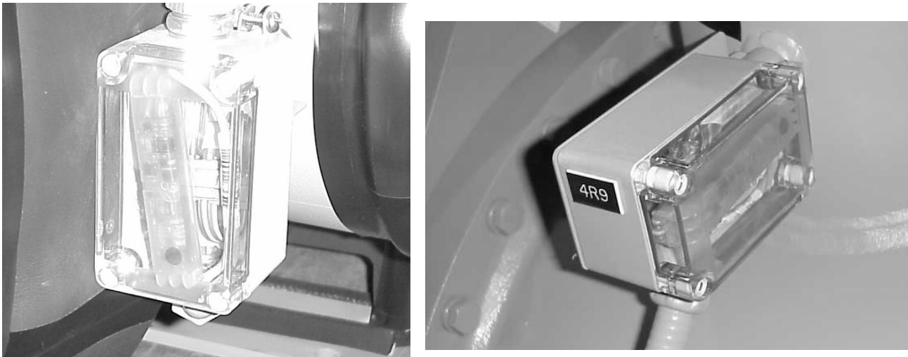
Figure 4 - Typical photographs of a temp sensor/polycarbonate box
