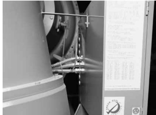
Figure 18. Control panel mounting bracket
