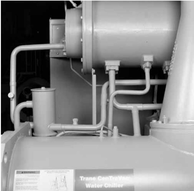
Figure 14. Lubrication system motor cooling lines
