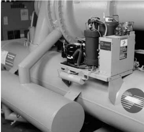
Figure 6. Purge unit detail
