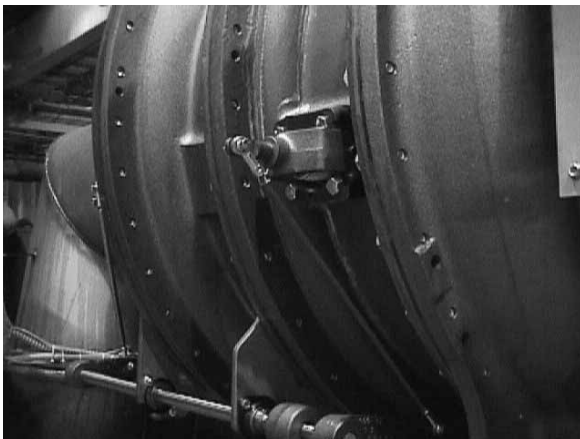
Figure 11. Vane actuator level on interstage
