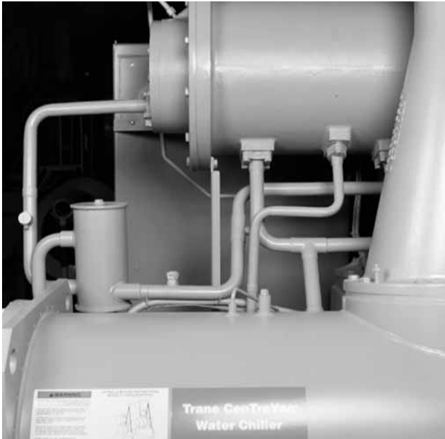
Figure 14. Lubrication system motor cooling lines
