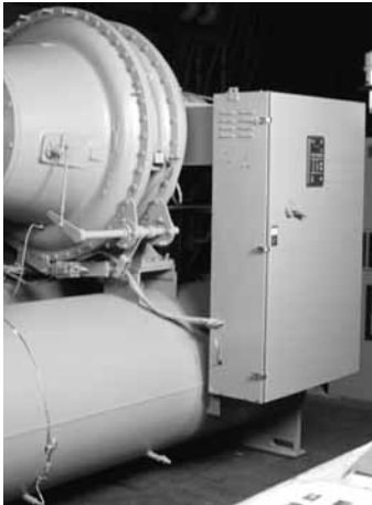
Figure 20. Starter mounting bracket
