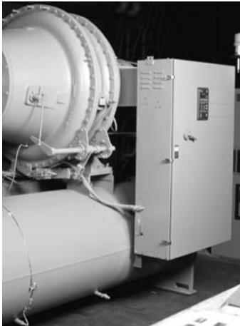
Figure 20. Starter mounting bracket
