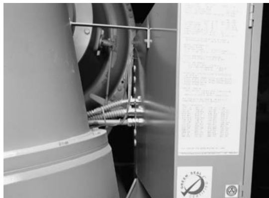
Figure 18. Control panel mounting bracket
