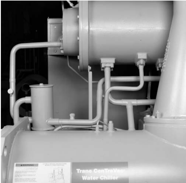
Figure 14. Lubrication system motor cooling lines
