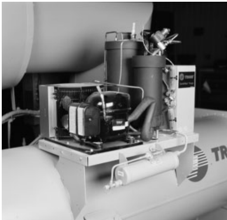
Figure 26. Purge unit details
