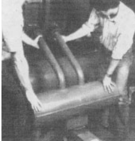
Figure 16. Removing the economizer
