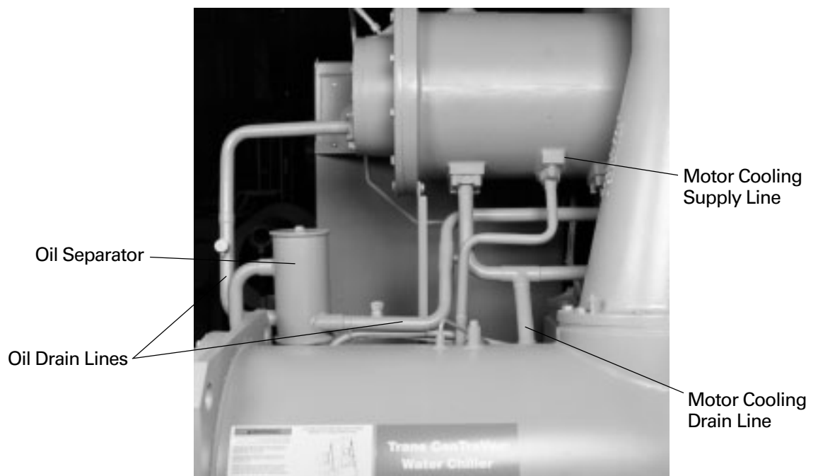
Figure 11. Typical motor cooling lines
