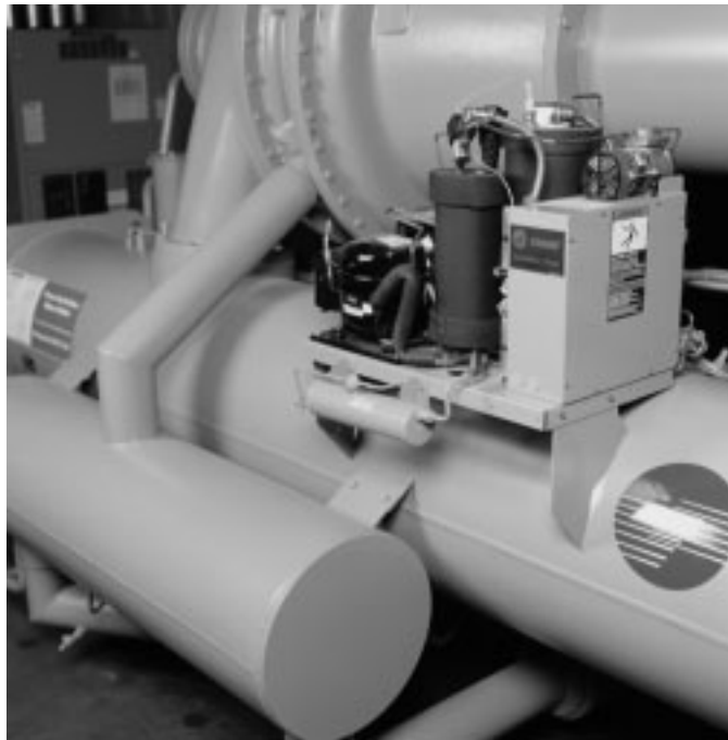
Figure 26. Purge unit details
