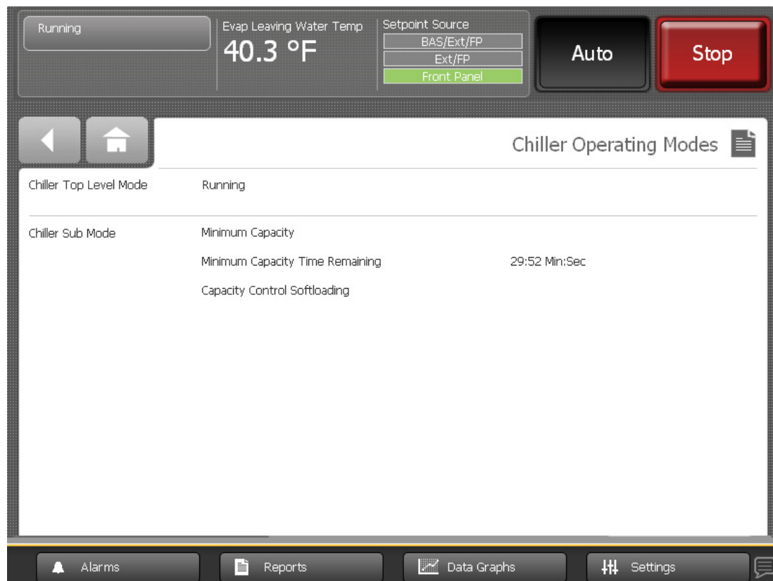
Figure 11. Chiller Operating Modes screen for CVHE, CVHF, and CVHG chillers
