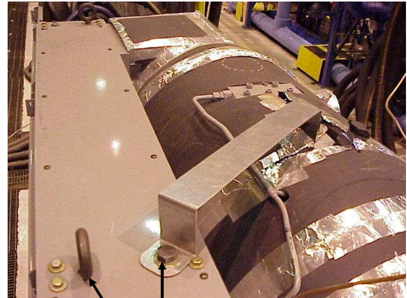
VFD Shipping Bracket
