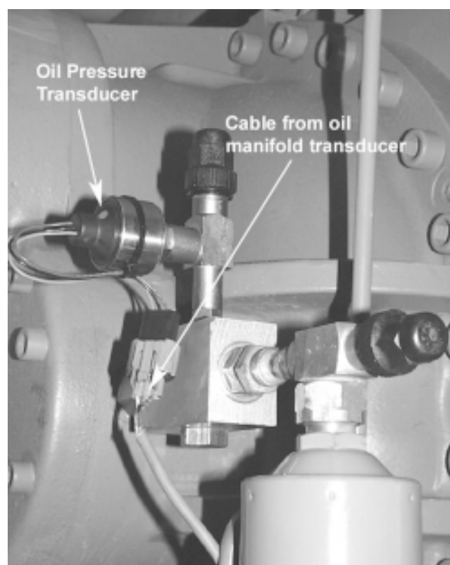
FIG. 24 – TRANSDUCER WIRING DETAIL
