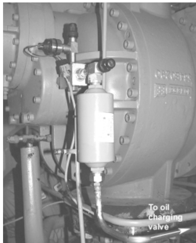
FIG. 23 – COMPLETE PIPING MODIFICATION, 233 mm
