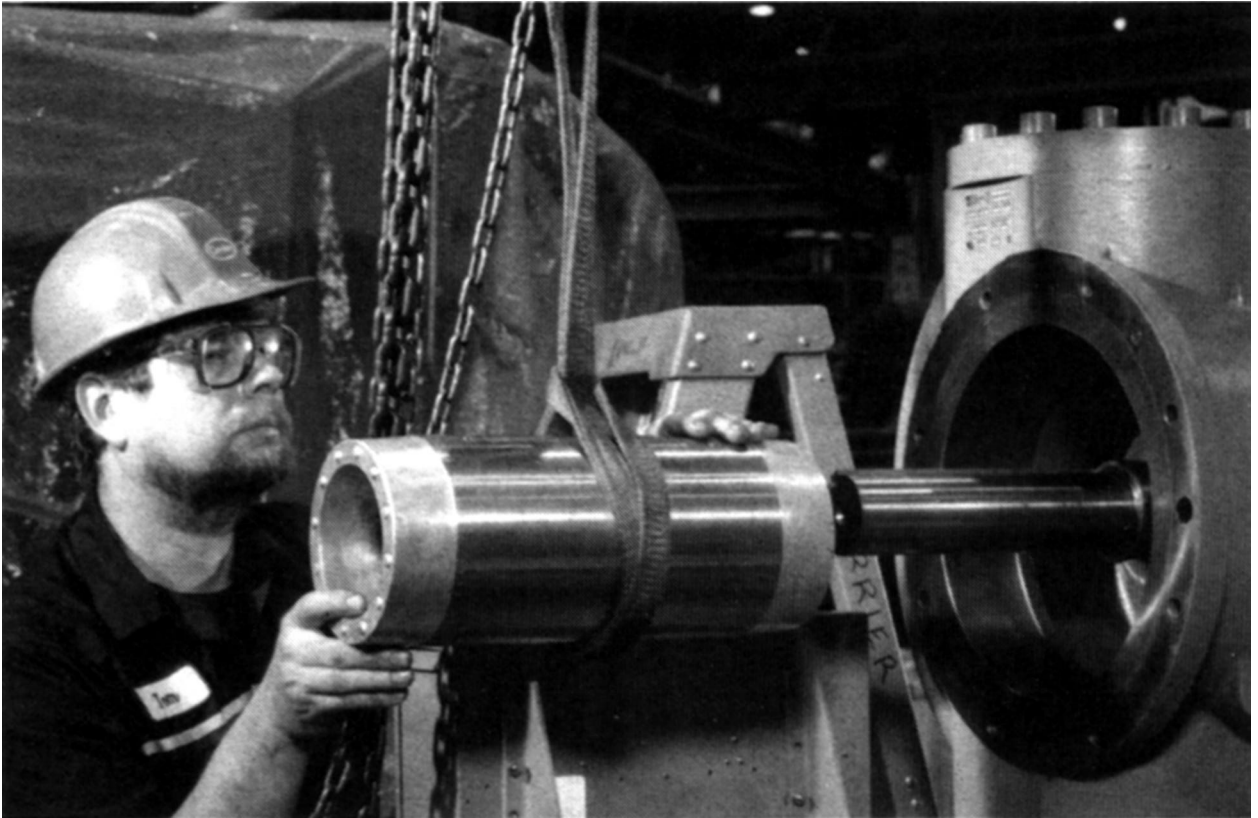
Figure 38 — Rigging the Rotor
