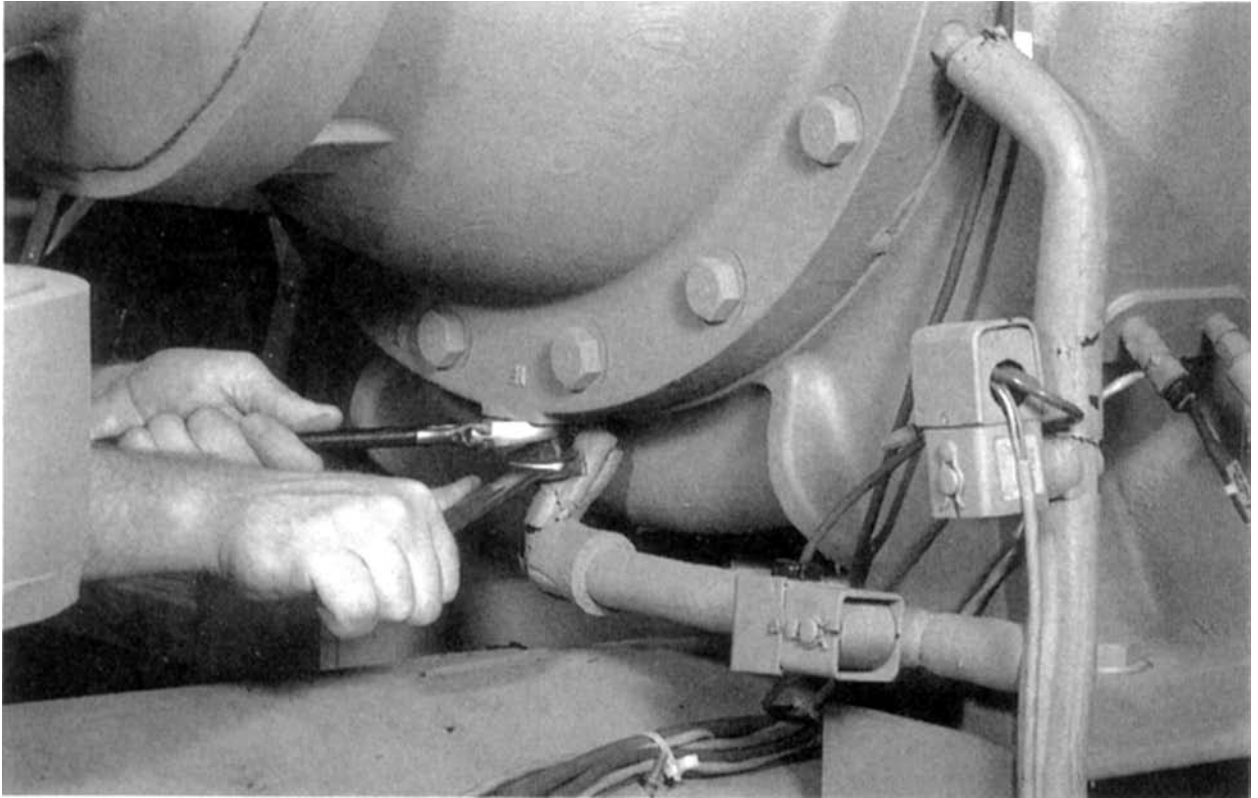
Figure 25 — Disconnecting the Oil Reclaim Lines
