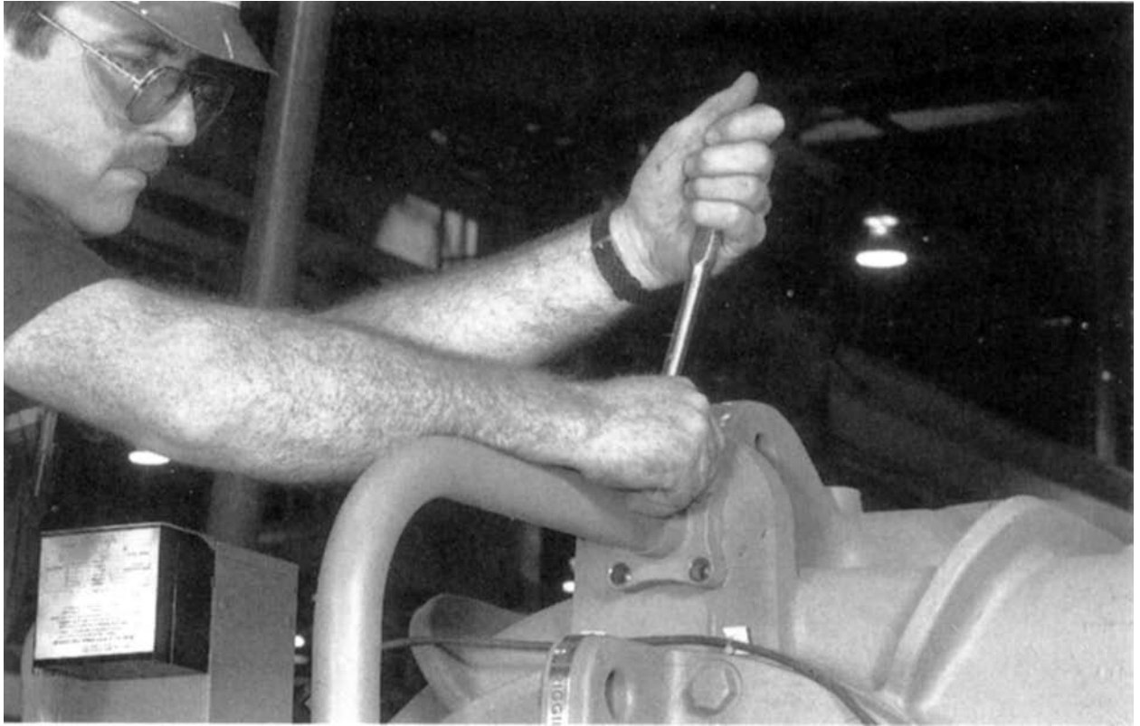
Figure 26 — Removing the Suction Ell
