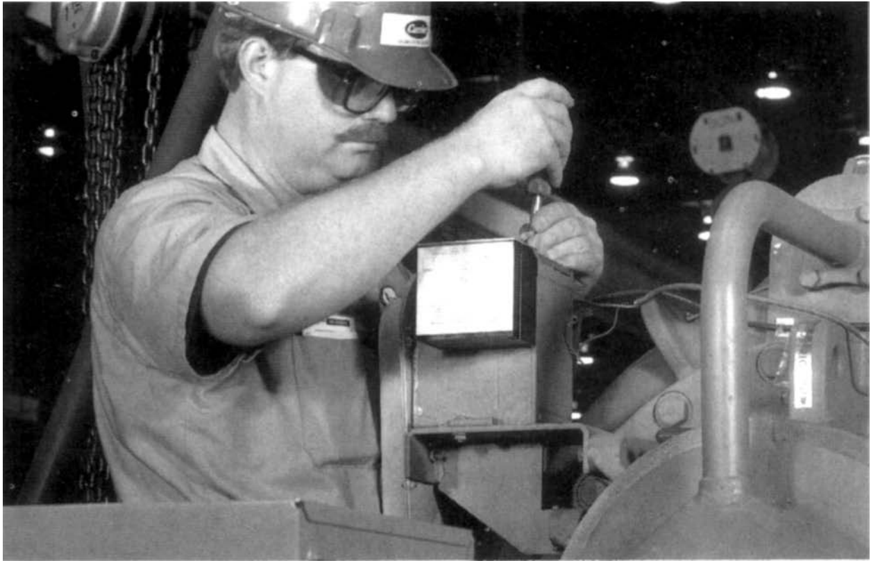
Figure 24 — Disassembling the Compressor
