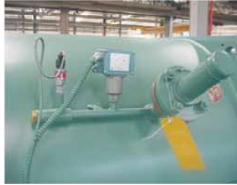
FIGURE 15 - RUPTURE DISK FROM FACTORY
