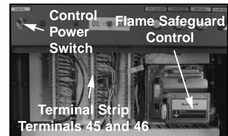
Fig. B17 Location of Terminals 45 and 46
