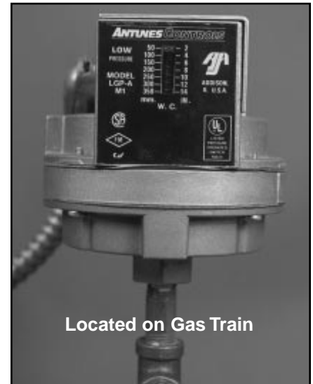
Fig. B16 Low Gas Pressure Switch
