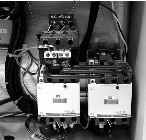
Fig 2.3 Typical Output Power Connection
