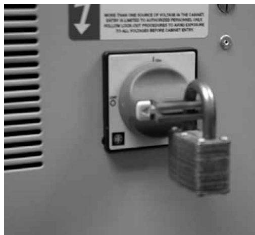
Fig 1.6 Disconnect Handle Positions – Shown OFF, With Padlock
