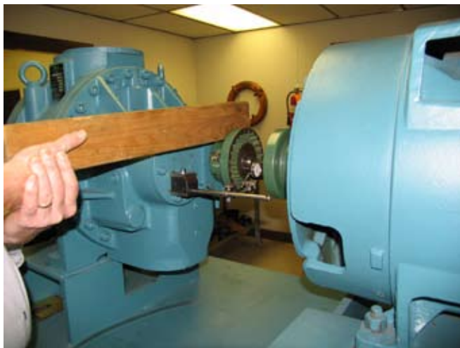
Figure 2. Board is positioned between the compressor and coupling to force the rotor towards the motor.
