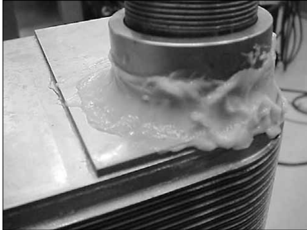
Figure 4 - Application of heat-sink paste before welding
