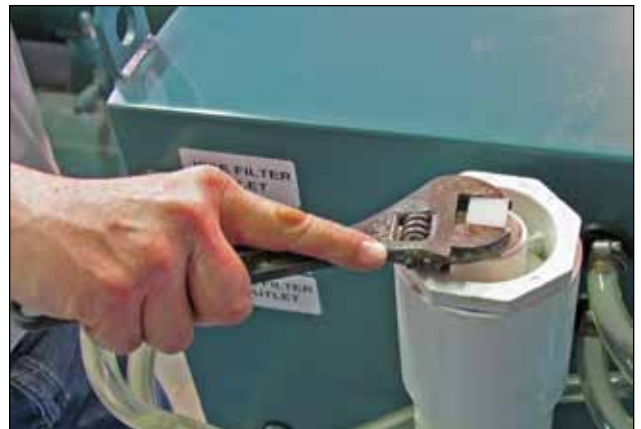
Figure 39 - Installing the Cooling System Pipe Plug
