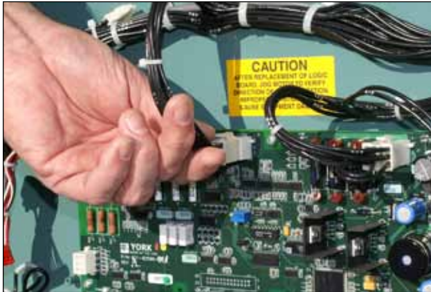
Figure 37 - VSD Logic Board Connection J2
