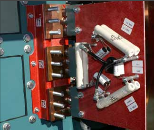
Figure 23 - Vyper™ Output Power Terminal Connection Lugs
