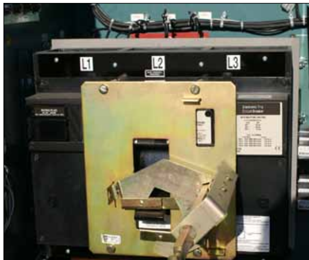
Figure 19 - Vyper™ Input Power Terminal Connection Lugs
