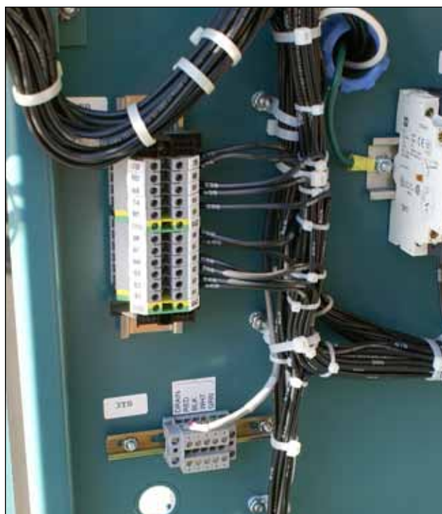
Figure 25 - Quantum™ LX Communications Terminal Block
