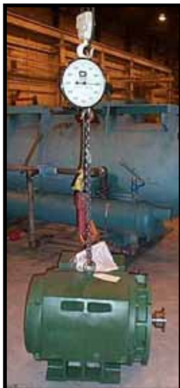
Figure 15. Weigh replacement motor
