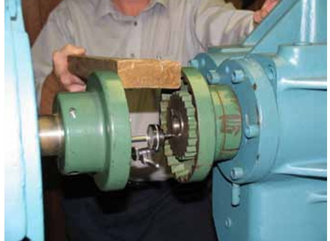
Figure 3 Board is positioned between both couplings to force the rotor towards the compressor.
