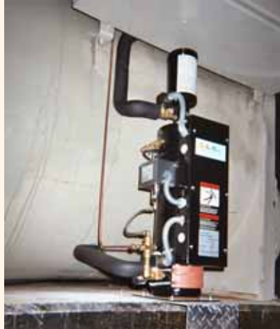
OAM-Purger installed at the University of Missouri.
