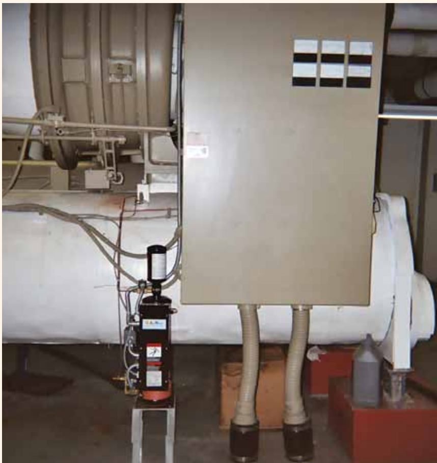
Professional Heating & Cooling, Inc. (Norfolk, VA.) Service Technician, Buddy Green, installed the OAM-Purgers at Norfolk Southern Towers.
