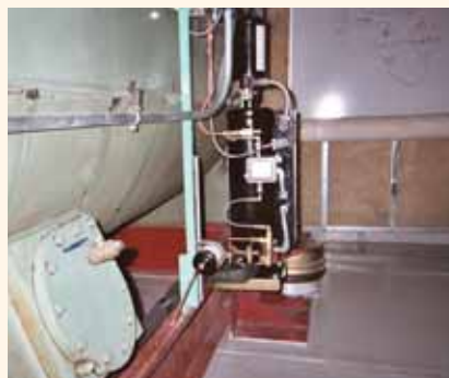
Ron Summerhays, Service Foreman, Johnson Controls (Anchorage, Alaska) installed OAM-Purgers at BP and Frontier Towers facilities.
