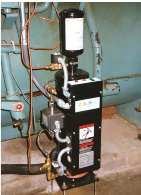
According to Redi Controls, its Industrial OAM-Purger can restore chiller capacity, thus offering substantial energy savings for building owners.
