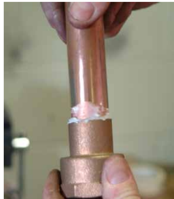
FIGURE 90 - SEATING PIPE TO FITTING
