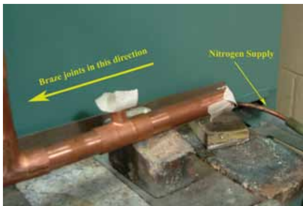
FIGURE 92 - BRAZING JOINTS IN DIRECTION OF FLOW
