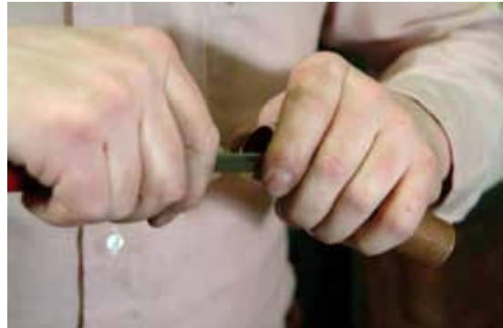
FIGURE 86 - CLEAN PIPE AFTER CUTTING AND BEFORE FITTING
