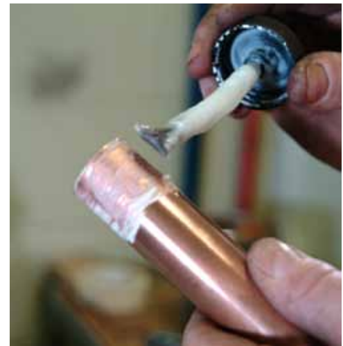
FIGURE 89 - APPLYING FLUX TO PIPE
