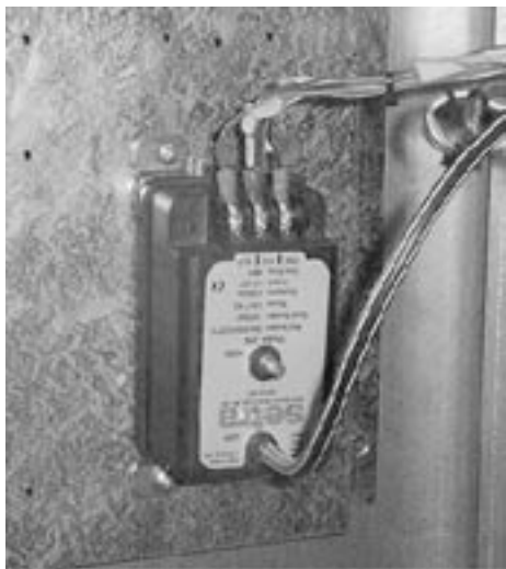
FIG. 2 – DUCT STATIC OR BUILDING STATIC TRANSDUCER
