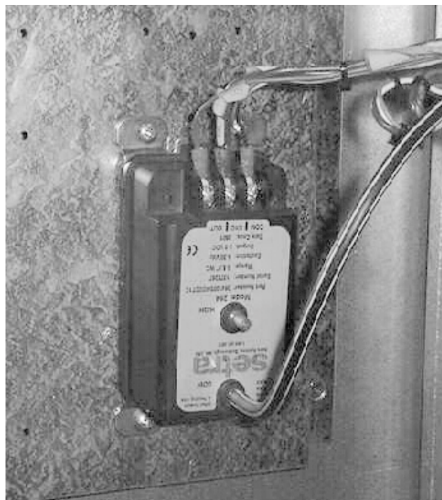
FIG. 2 – DUCT STATIC OR BUILDING STATIC TRANSDUCER (LOCATED IN RETURN SECTION OF UNIT)
