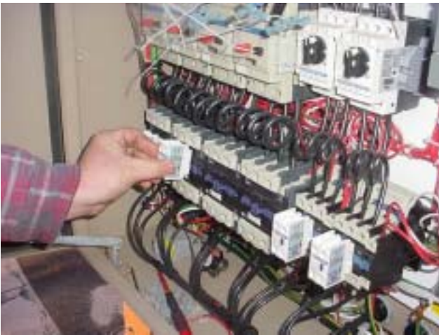
FIG. 13 - INSTALL TOP MOUNT AUXILIARY CONTACTS
