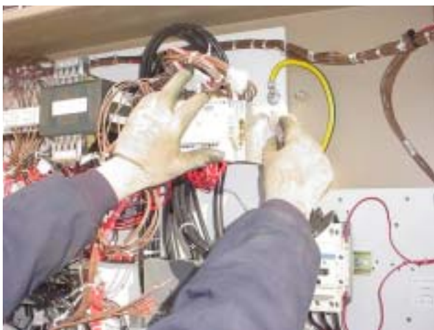
FIG. 8 - MARKING SMART RELAY BRACKET HOLE LOCATIONS
