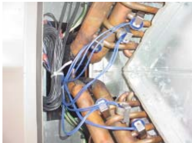
FIG. 23 - FINAL FREEZESTAT WIRING (6-COMPRESSOR UNIT SHOWN)
