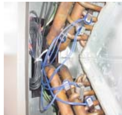
FIG. 18 - ROUTING FREEZESTAT WIRING FROM CONTROL PANEL TO COIL HEADER
