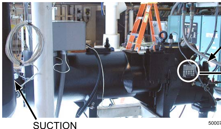
FIG. 8 - Check Pressure At Port
