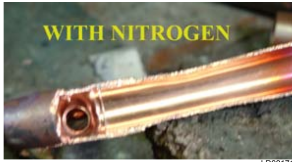
FIG. 7 - PIPE BRAZING WITH NITROGEN
