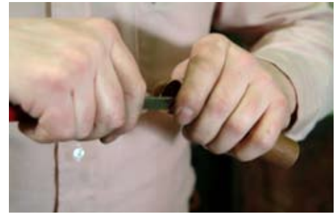
FIG. 9 - CLEAN PIPE AFTER CUTTING AND BEFORE FITTING
