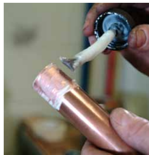
FIGURE 89 - APPLYING FLUX TO PIPE
