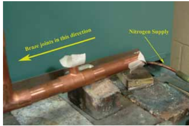
FIGURE 92 - BRAZING JOINTS IN DIRECTION OF FLOW
