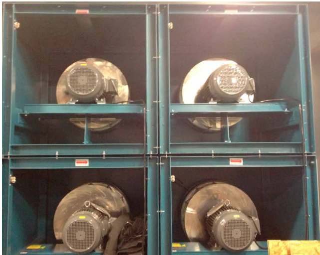
FIGURE 9 - BACK OF A 2X2 FAN ARRAY
