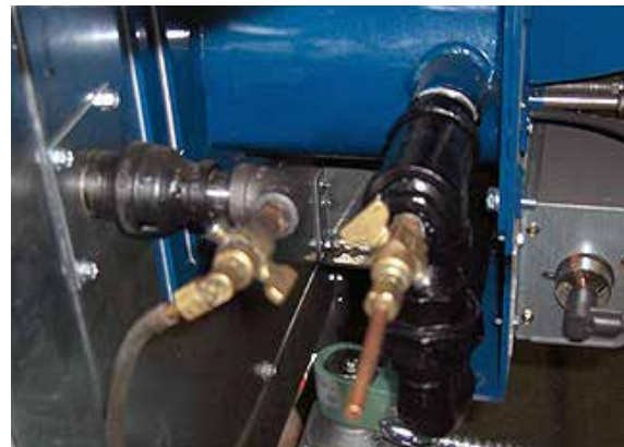
FIGURE 32 - DRAFT OVER FIRE TEST PORT
