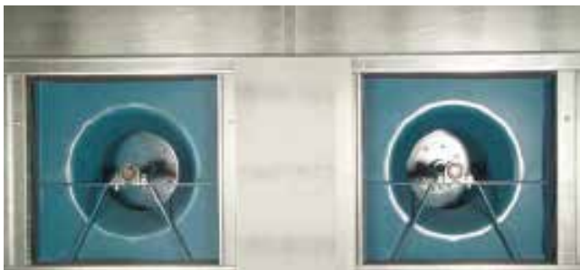
FIGURE 10 - FRONT OF A 1X2 FAN ARRAY
