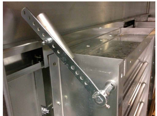
FIGURE 7 - COUNTERBALANCE UNLOCKED FOR START-UP
