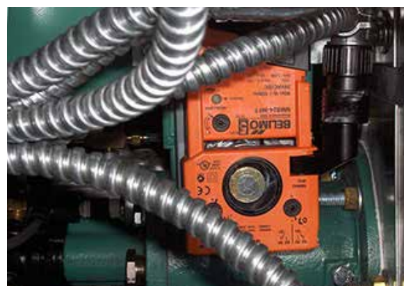
FIGURE 34 - DAMPER ACTUATOR
