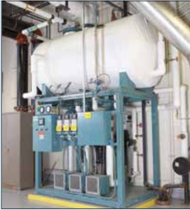
The deaerator uses a mechanical scrubbing method to eliminate the harmful gases from a feedwater supply.
