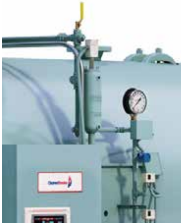
Figure 1-27: Water Column and Vent Valve
