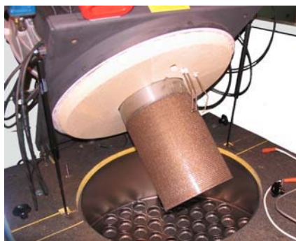
Figure B5-2. Fireside Access
