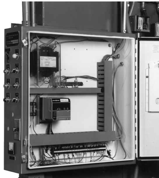
Fig. 14. Electrical panel installation.
