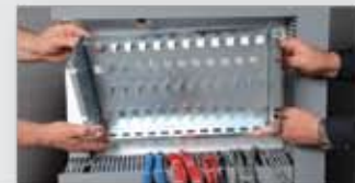
Install the I/O conversion base plate in the control panel. Attach conversion base plate.
