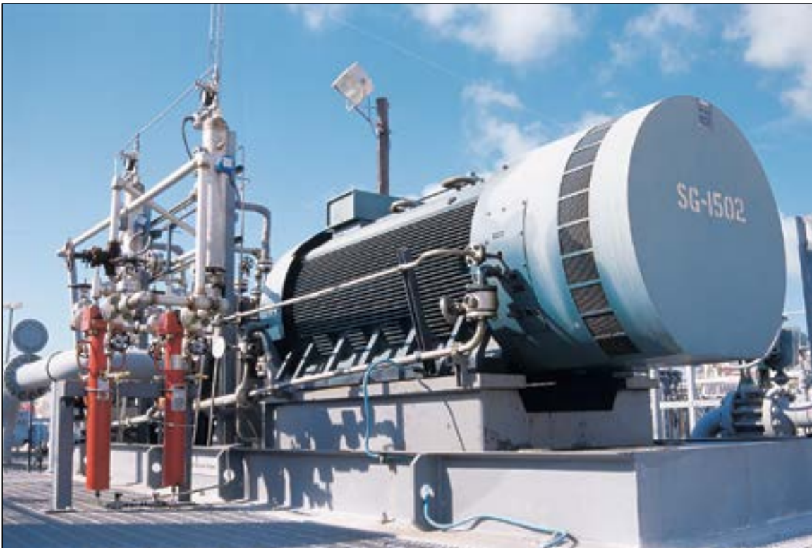
This is an API 541 TEFC G500M motor operating a compressor in a petroleum refinery.
